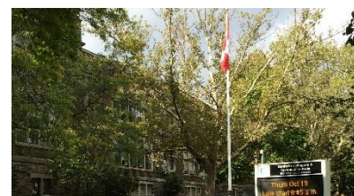
Greenwood Secondary School
